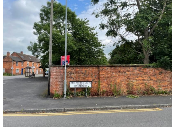
Plate 5: Western boundary of the Site.
