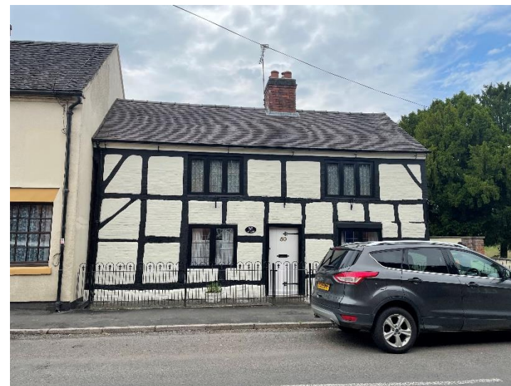
Plate 33: Rose Cottage as seen from the High Street.
