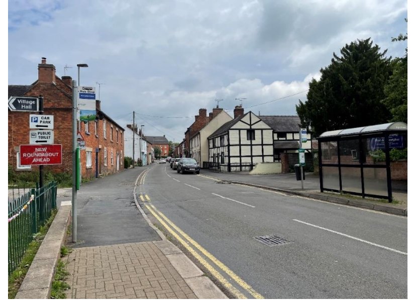
Plate 19: View east opposite the Site demonstrating the set back to the north and south of the High Street.
