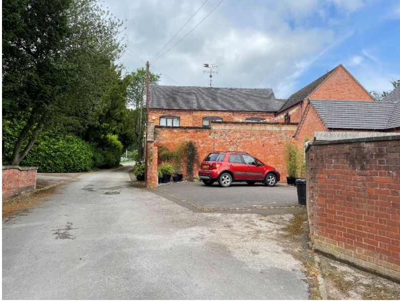
Plate 30: Converted ancillary buildings and remnants of the historic drive.
